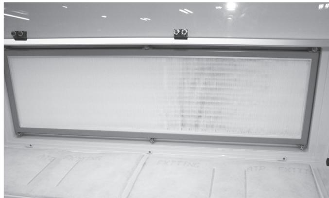
**Figure 9. AC740C Pre-filter and HEPA filter.**
